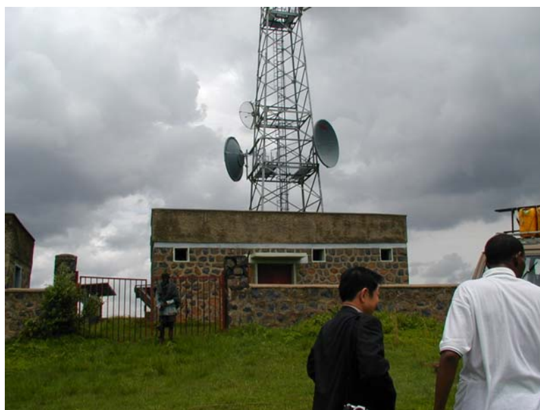
Merawi PCO Base Station (Planned Construction site)
