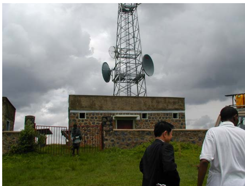
Attachment – 8 Merawi PCO Base Station (Planned Construction site)
