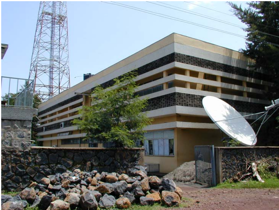
Attachment – 1 Bahir Dar Region Primary Center (P.C.) (Central Building external appearance)
