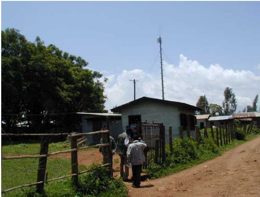
Attachment – 4 Woreta City Station (ETC Tele-house in front, DRMASS Antenna in back side)
