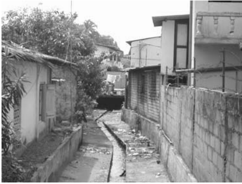
5-19 View of upper reaches of Nugegoda Ela in Kohuwala The channel is lined with concrete. Photo was shot from culvert near proposed upstream end of channel improvement.
