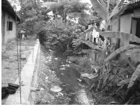
5-13 View of upper reaches of Delkanda Ela near upstream end of channel improvement Photo was shot from left bank to downstream.
