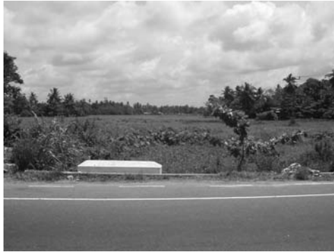
5-8 View of upper reaches of Katubedda Tributary Photo was shot from Piliyandala Road Culvert to downstream.
