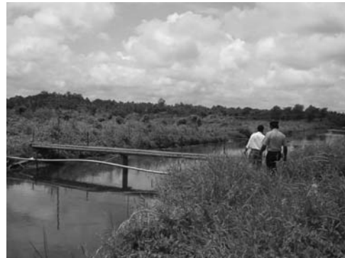
5-12 View of lower reaches of Bolgoda Canal along Sri Lanka Air Force Base Photo was shot from right bank to downstream.
