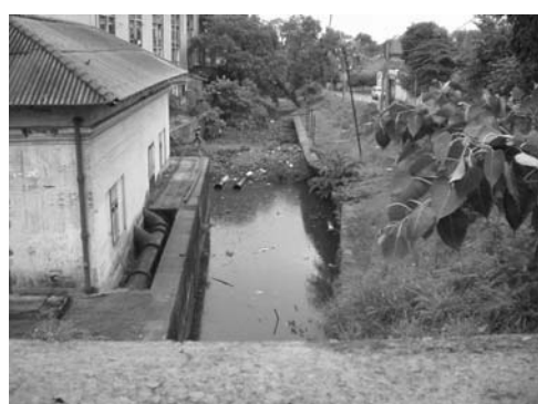
3-6 View of St. Sebastian Canal pumping station Photo was shot from St. Sebastian Hill Road Bridge to Beira lake side.
