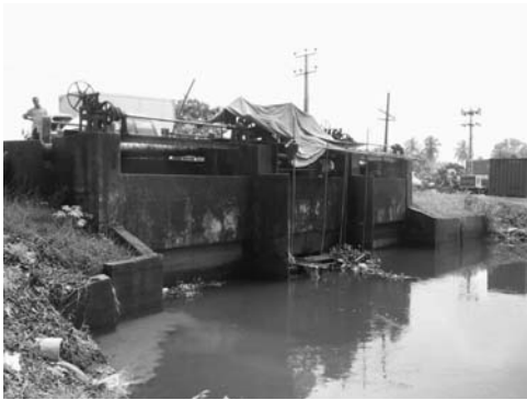
2-2 Downstream view of existing Wattla Gate at Hekitta Road Bridge
