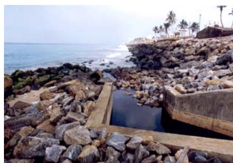
Photo 6 Unity Place Scheme Outfall -November 2001-
