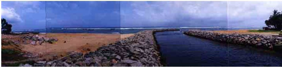
Photo 7.21 Dehiwala Outfall -July 2002-
