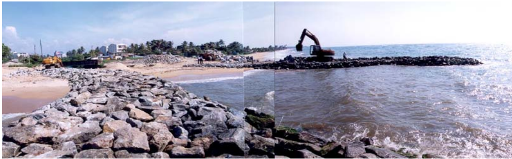
Photo 10 Dehiwala Outfall (Under Construction) -November 2001-
