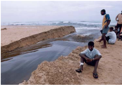
Photo 7.13 Lunawa Lake Outfall (Just After the Breach) -November 2001-
