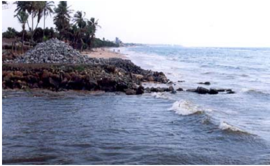
Photo 8 Wellawatta Outfall (South) -November 2001-
