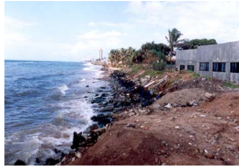
Photo 9 Wellawatta Outfall (North) -November 2001-
