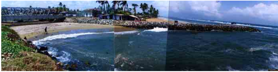
Photo 7.20 Wellawatta Outfall -July 2002-
