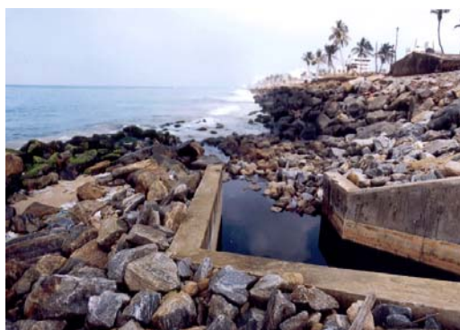
Unity Place Outfall
