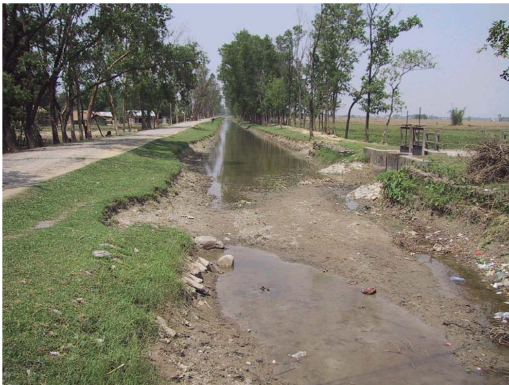
Shankarpur Canal at a mid-stream part. The condition is better than Suksena Canal since it was once rehabilitated under Stage I of SMIP. However, the water delivered is not enough to cover the planned area due to sandy soil prevailing in the Study area.
