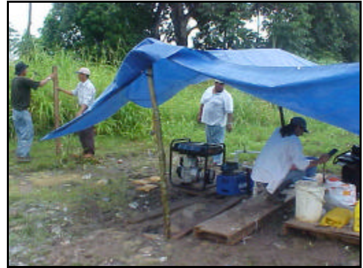
Photo 2. Well #6 work area.
