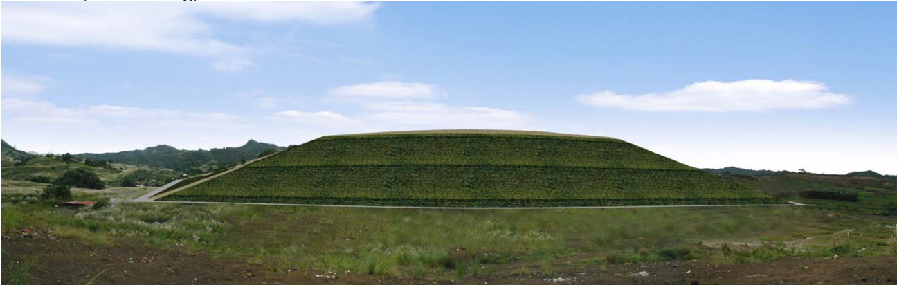
Phase 4 (after filling)
