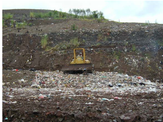
2) Heavy equipment fully compressed waste
