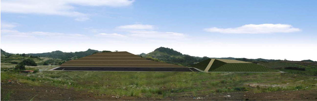
Phase 2 (before filling)
