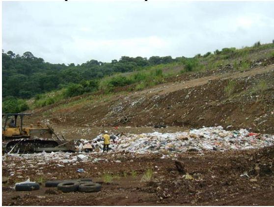
1) Waste was placed within a specified working area
