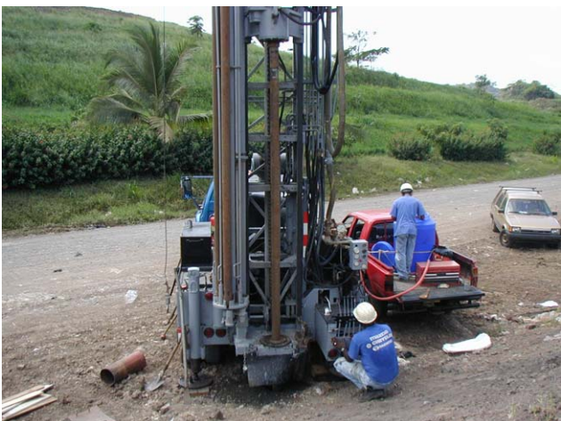
Well construction for sampling groundwater
