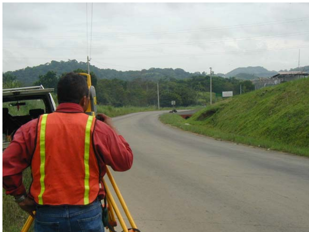
Topographic survey was conducted by using total stations
