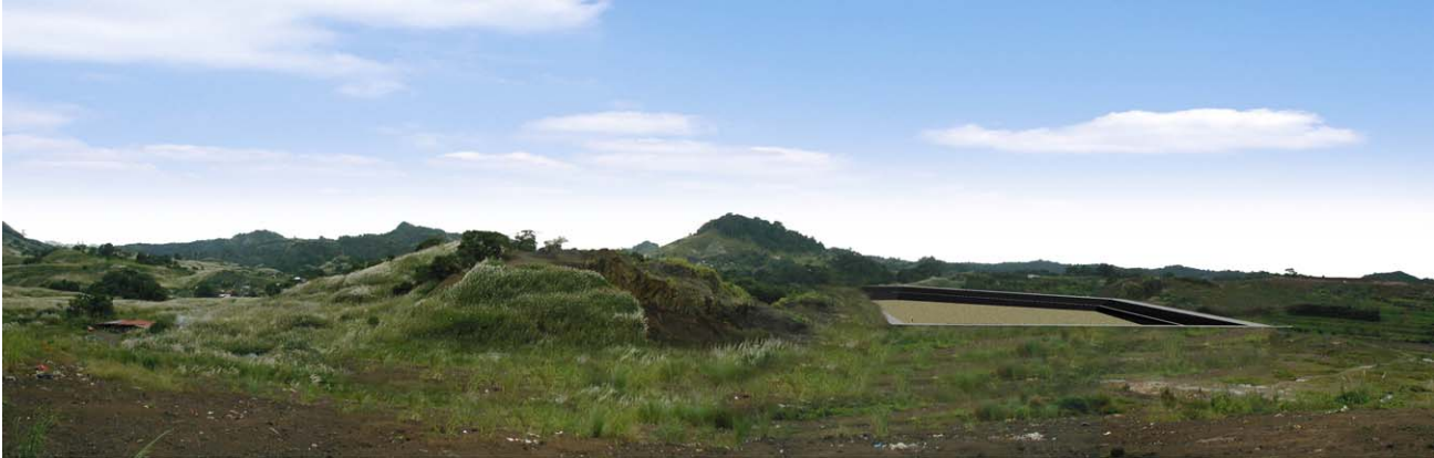
Phase 1 (before filling)
