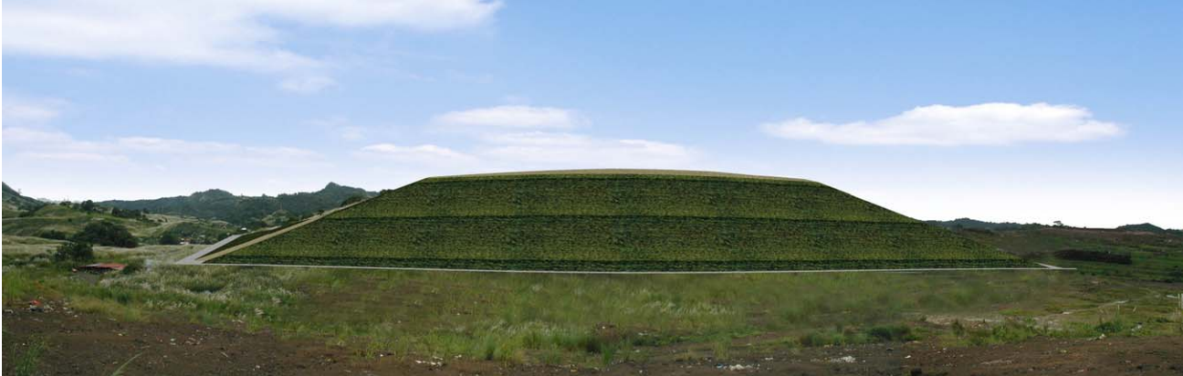
Phase 4 (after filling)
