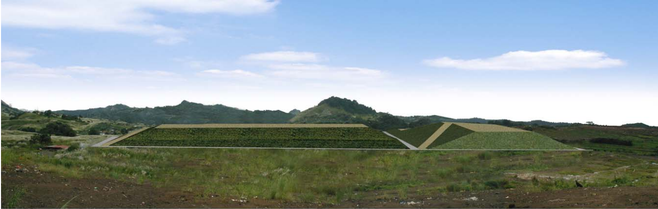
Phase 3 (before filling)
