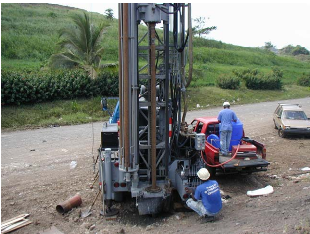
Well construction for sampling groundwater
