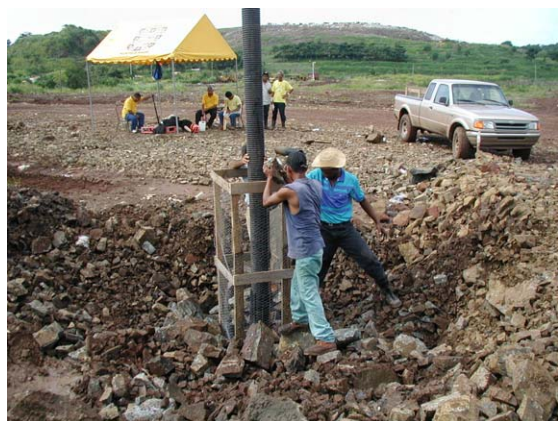
Installment of landfill gas extraction pipe
