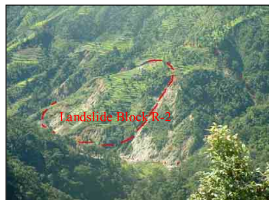
Landslide R-2 of 1.5km upstream from Regulating Pond
