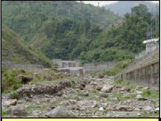
KL-II P/S (Above-ground)
