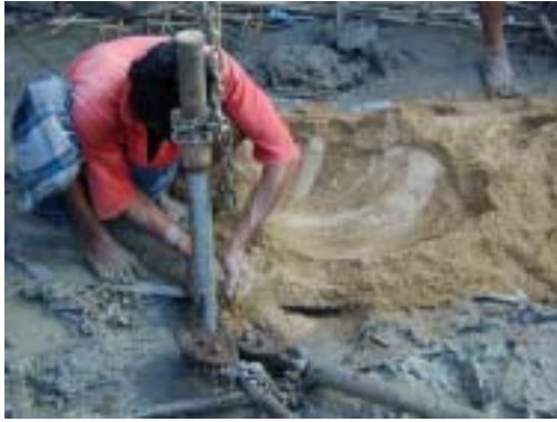
a) Coarse sand filling
