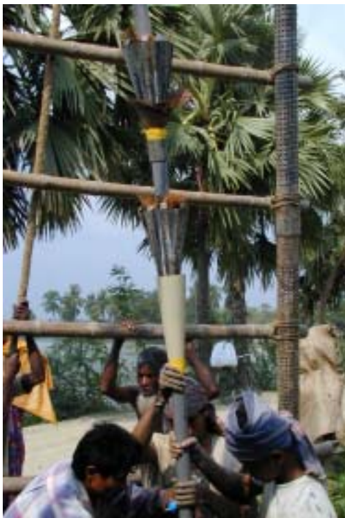
Figure 5.15 Inner of Metal-petal-basket
