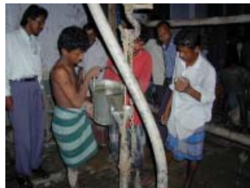
e) Cement milk injection
