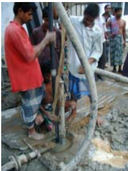
c) Tremie pipe incertion
