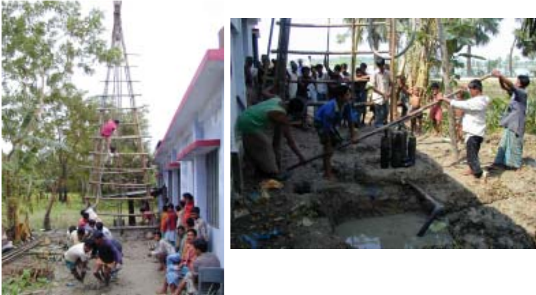
Figure 5.8 Drilling by Donkey method
