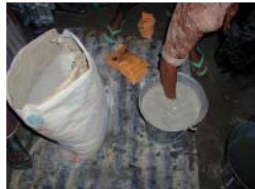
d) Cement milk making
