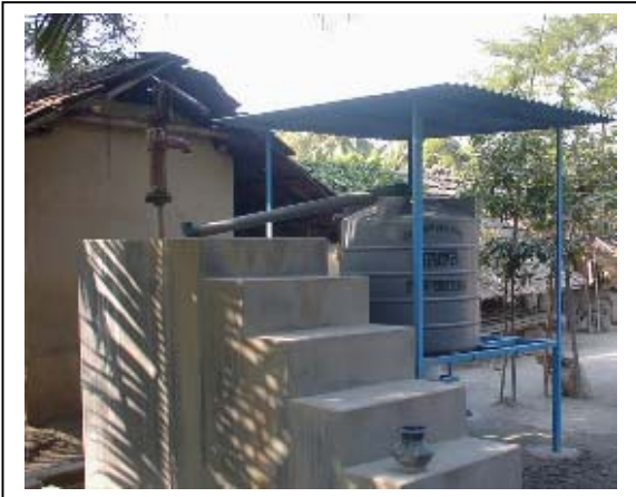
Before and after installation. Site for passive sedimentation unit (PS3) I.D. No. ? Tube well no. TW-23
