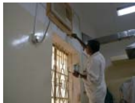
Installation of air conditioner
