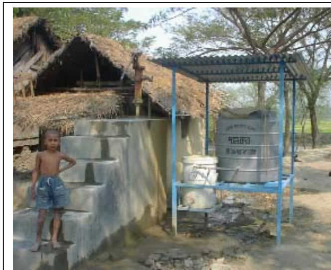
After construction of platform and installation of passive sedimentation unit (PS1)
