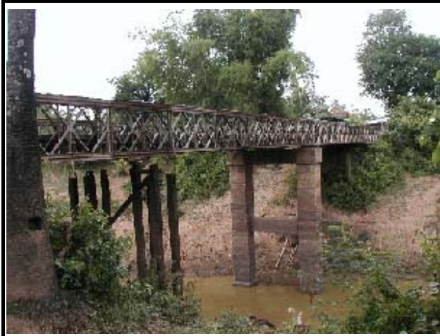
Side View of Existing Bridge
