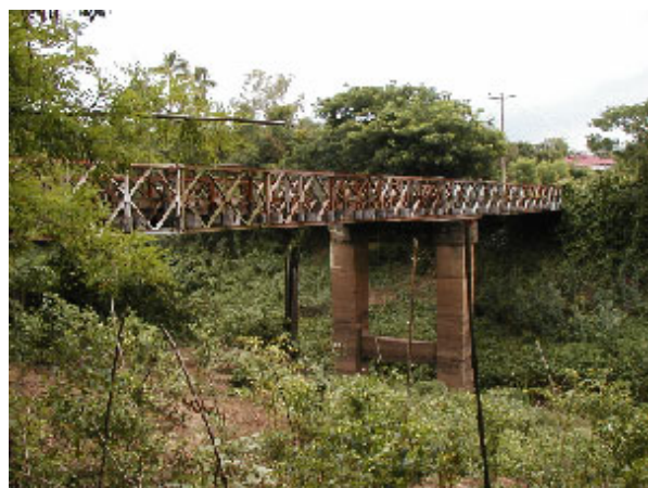
Side View of Existing Bridge
