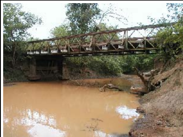
Side View of Existing Bridge
