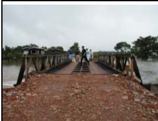
View from Left Bank to Right Bank
