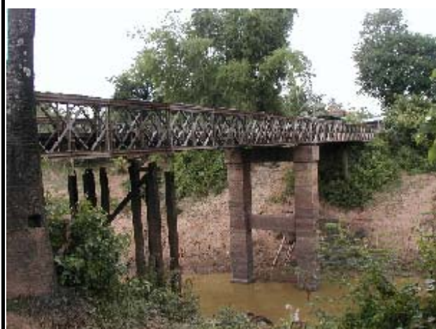
Side View of Existing Bridge
