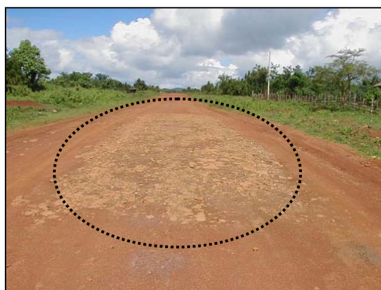
Figure 1.2.26 Damaged Surface – Ravelling ( at 8.9km )
