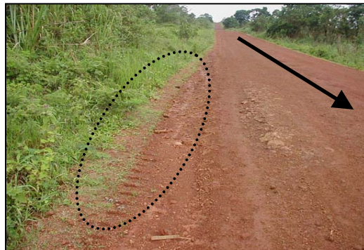
Figure 1.2.24 Damaged Surface – Rutting ( at 2.0km )
