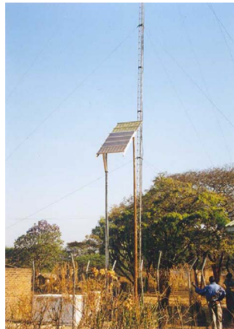
Photo 8-10 Post Office with Solar Home System for Radio Telecommunication System (Bulala TC in Mzimba District)
