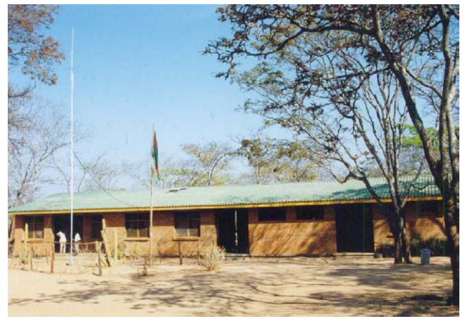
Photo 8-6 Hospital with Solar Home System (Mbalachanda TC in Mzimba District)
