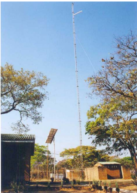
Photo 8-11 Telephone Office with Solar Home System (Mbalachanda TC in Mzimba District)
