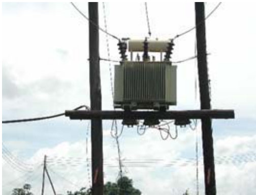
Fig. 5-1-8 Transformer (100kVA)
