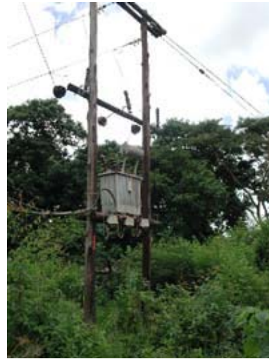
Fig. 5-1-7 Transformer (50kVA)
