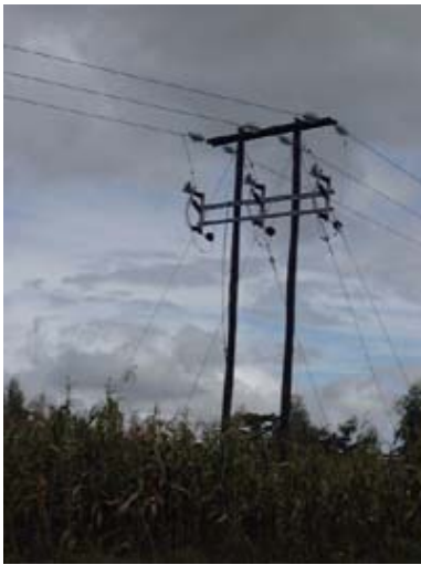
Fig. 5-1-3 Disconnecting Switch
