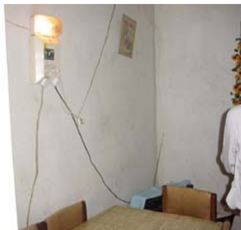
Fig.5-7-7 Ready Board and Wiring
