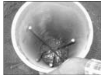
Setting of stone pillar
