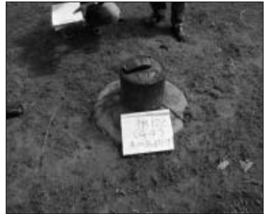
Existing control point (Close-range view of PM point)
