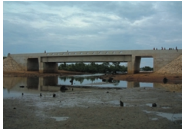
The constructed bridge on a trunk road (Mkindani bridge)
