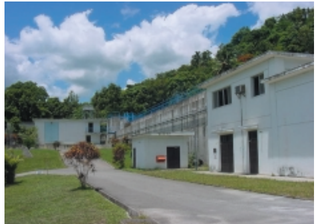
Water treatment plant of Santa Ana
