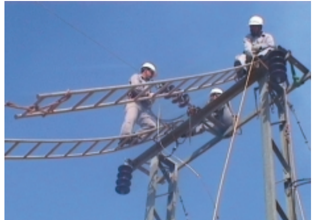
Training on the maintenance of transmission lines
