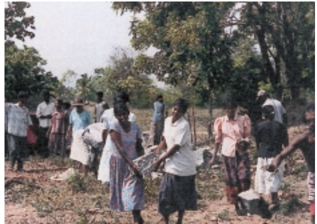
Building of an agricultural reservoir (cooperation of villagers)
