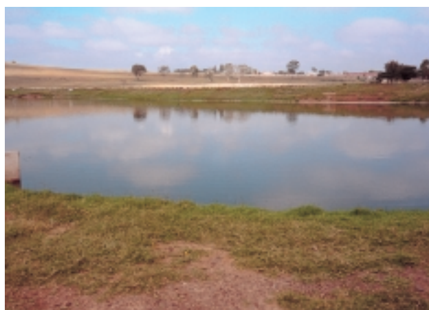
Sewage disposal facility in Nakuru District
