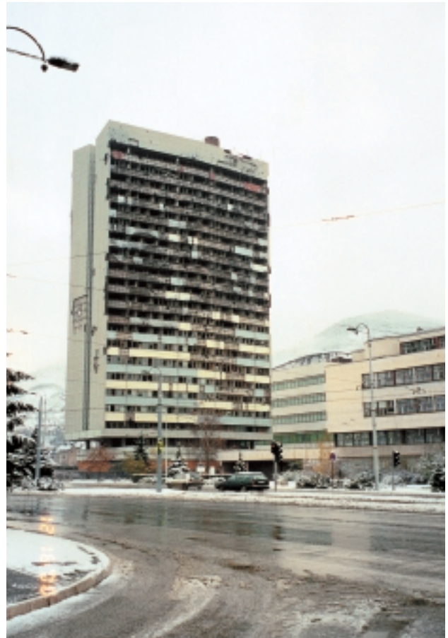
Building in downtown Sarajevo that remains in a state of disrepair
