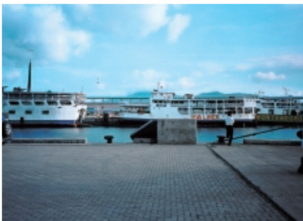
The Batangas Port (Passenger ship terminal)
