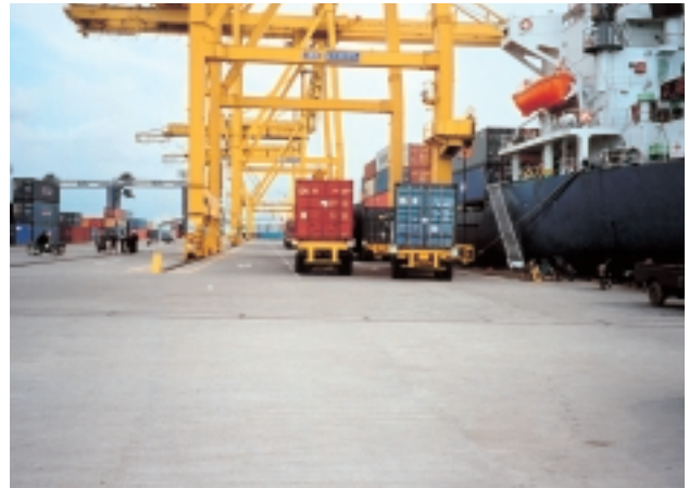
Container Terminal of the Port of Semarang
