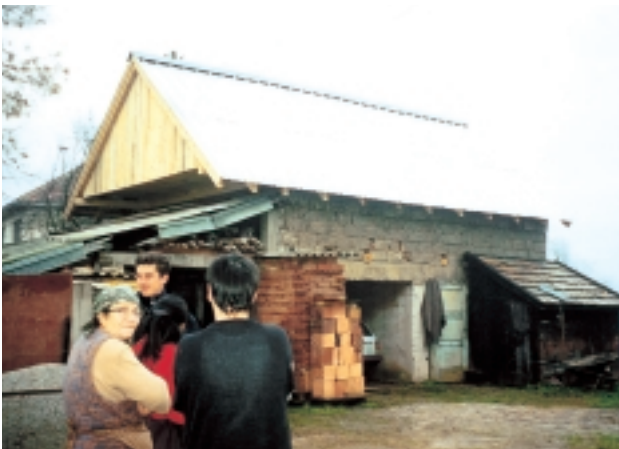
Repairing livestock shelters.
