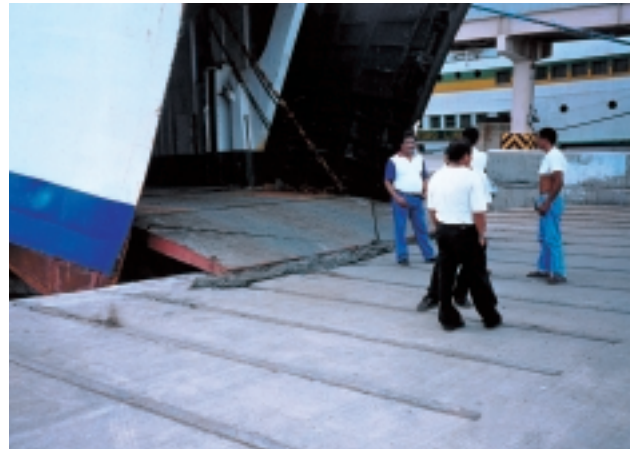
The Batangas Port (Ro/Ro ferry terminal)
