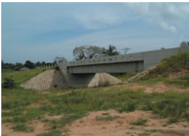
Mpapura bridge (Project for Improvement of Bridges on Trunk Roads)
