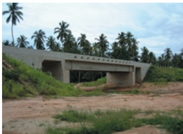
Mbuo bridge (Project for Improvement of Bridges on Trunk Roads)
