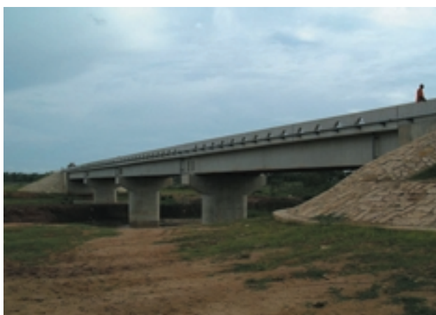
Mkwaya bridge (Project for Improvement of Bridges on Trunk Roads)
