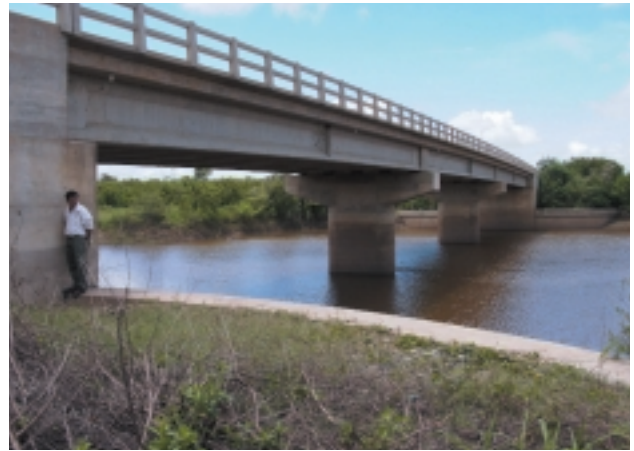
"Construction of Bridges in Northern Department of Santa Cruz" (Okirawa Payrón Bridge)
