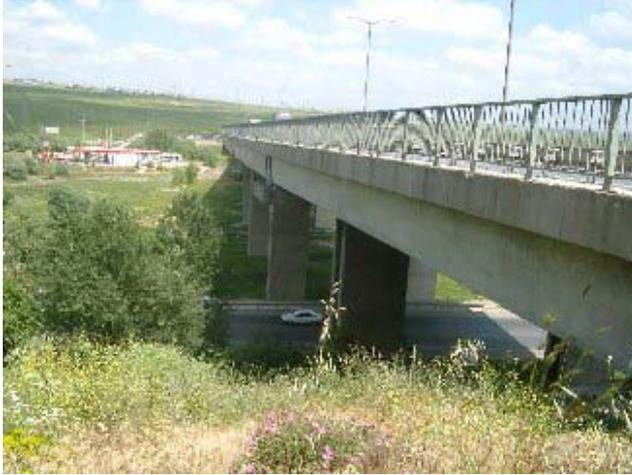
The evaluated result of this bridge is 89.8. The reason why this bridge possesses the high value is that this bridge is composed of simple beam of the girder and that pier is comparatively high. The collision between each girder can cause contingent boost of displacement and falling-off of the girder.
