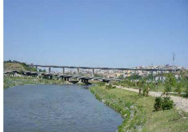
The evaluated result of this bridge is 79.2. The reason why this bridge possesses the high value is that this bridge is composed of simple beam of the girder and that pier is comparatively high.
