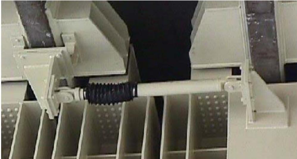
**Figure 9.5.6** An Example of Displacement Controlling by Damper
