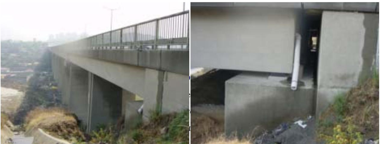
However the void between the girder end and the face of abutment is comparatively large, so there may not be a collision in this part.
