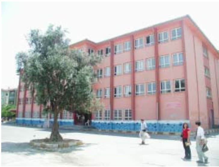
Photo 9.2.1 Primary School: Large Floor Area (A) to Height (H) Ratio
