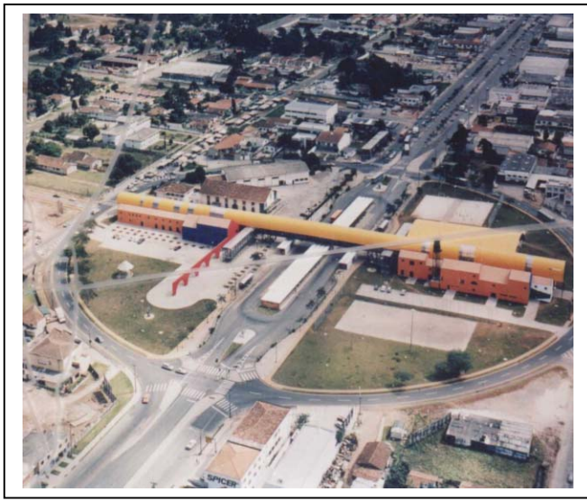
Figure 5.35 Busway Terminal, Curitiba, Brazil
