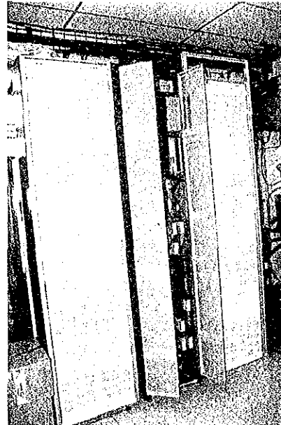
2-2 7Ghz/16Mbps Spur Microwave System installed in Luangprabang telephone office
