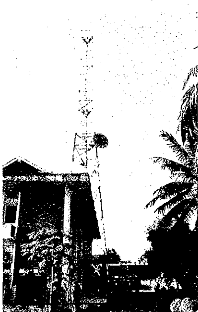
2-3 Microwave parabolic antenna and tower installed in Luangprabang telephone office
