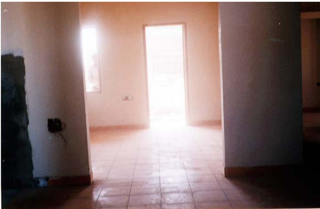
FLOORING WORK – C1 TYPE STAFF QUARTERS (18/01/02)
