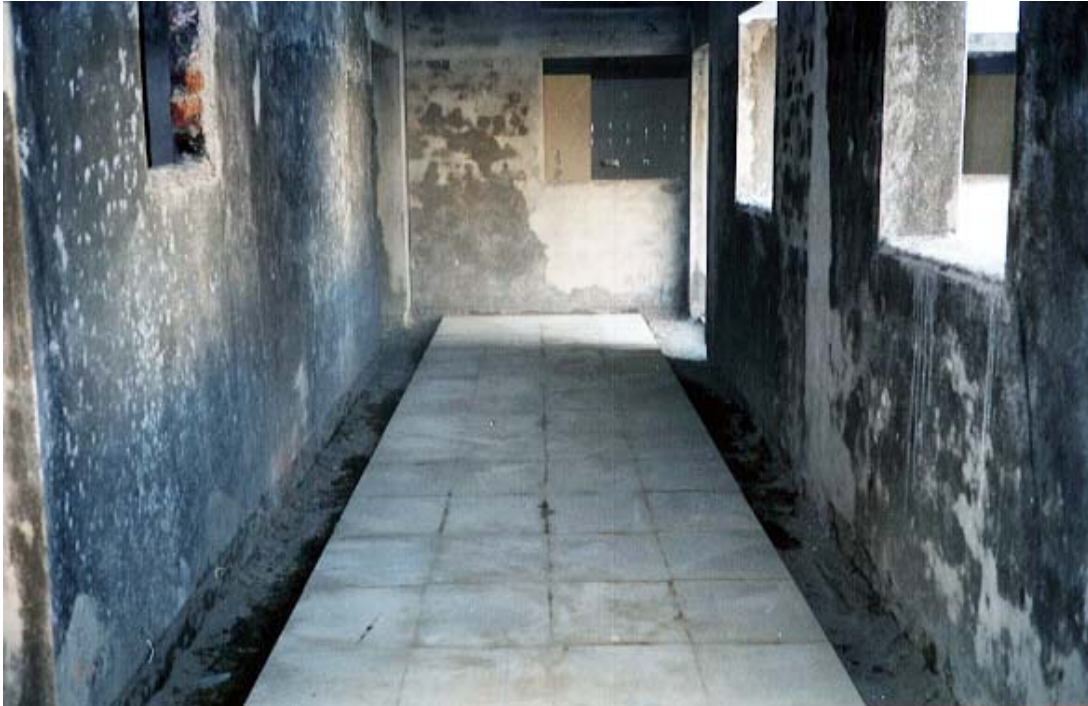
KOTA STONE FIXING – MAIN HOSPITAL (24/01/02)
