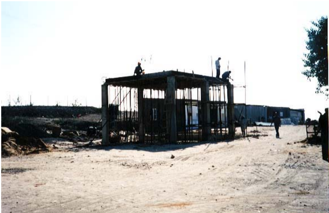
ROOF SLAB PREPARATION FOR AMBULANCE ROOM / D G ROOM (31/12/01)
