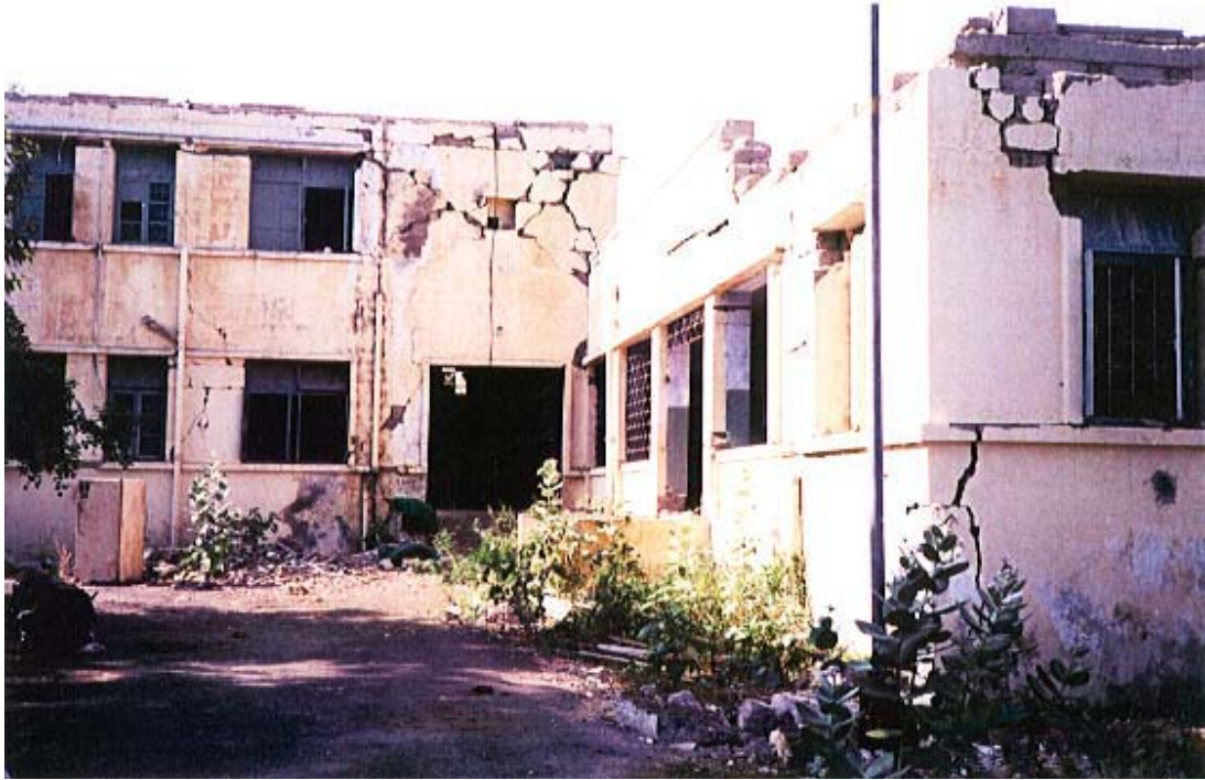
MAIN HOSPITAL BUILDING
