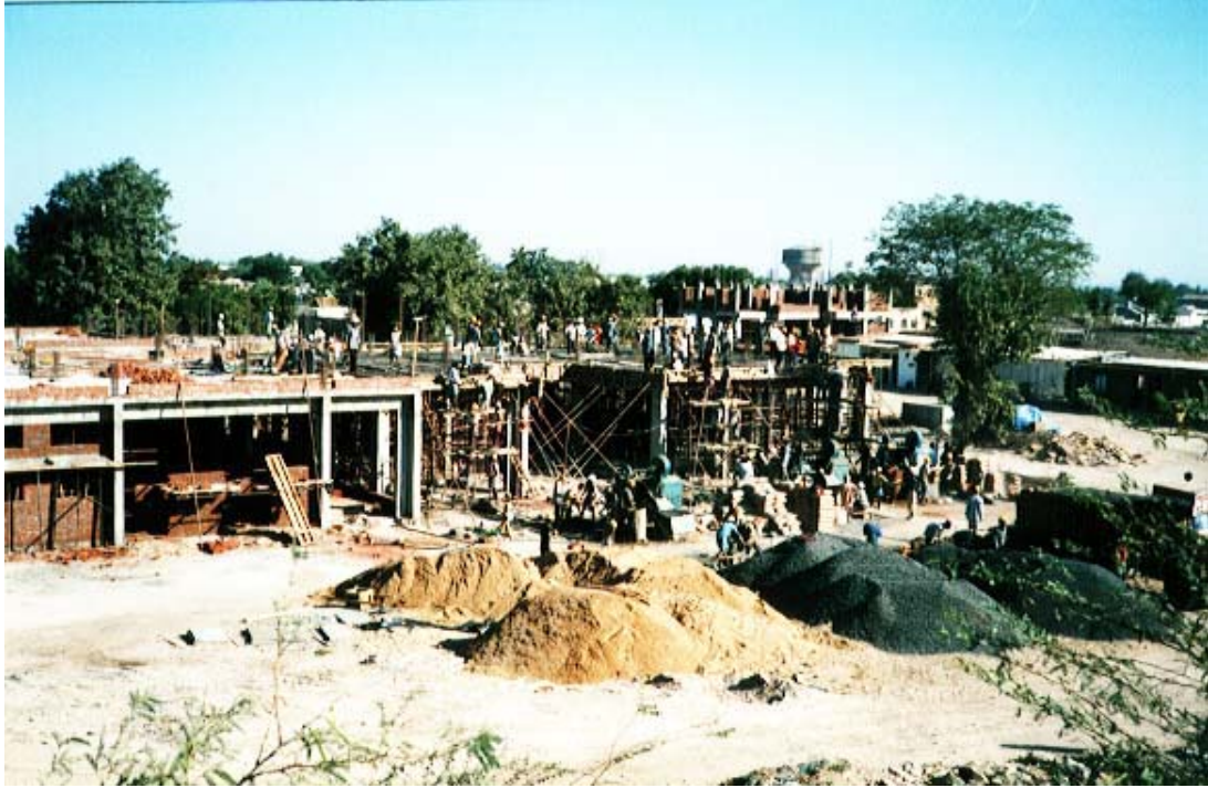
ROOF SLAB CASTING IN BLOCK 3 (07/12/01)
