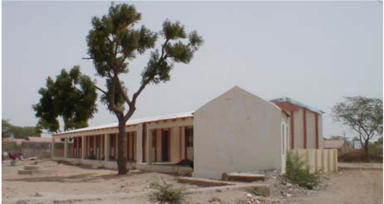
Sumarasar Sheikh Primary School Overall View (17/05/2002)
