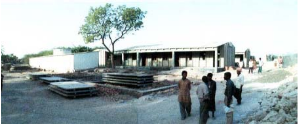
Bhadreshwar Primary Schools Overall View from Boys' School Side (27/03/02)
