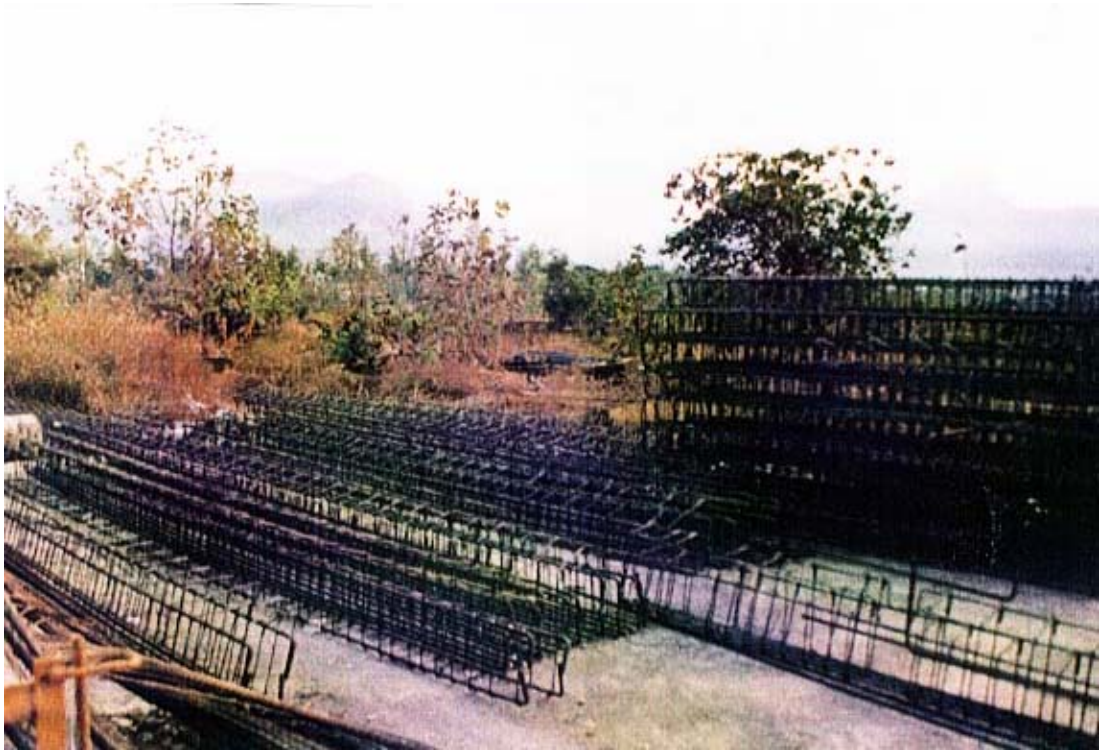
Beam Reinforcements as on 26/12/01
