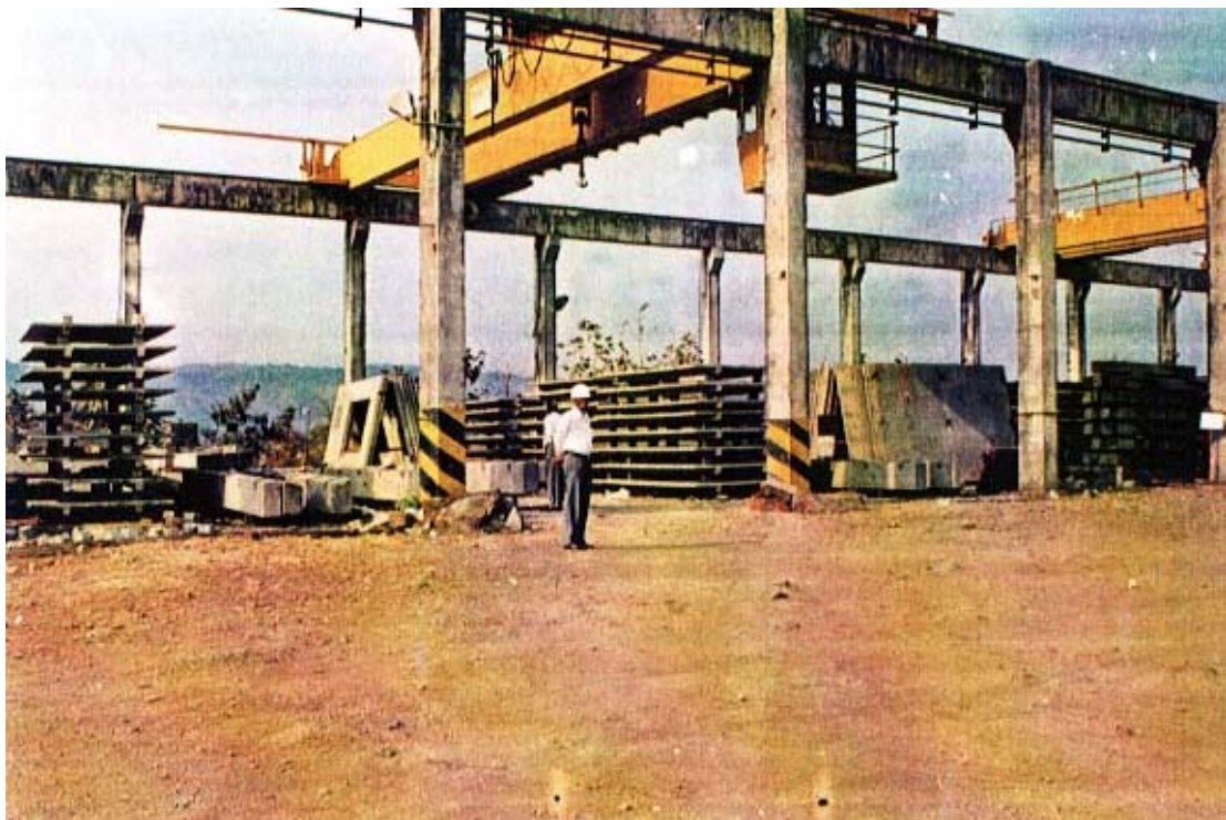
Stacking & Delivering Of Wall Panels as on 20/12/01
