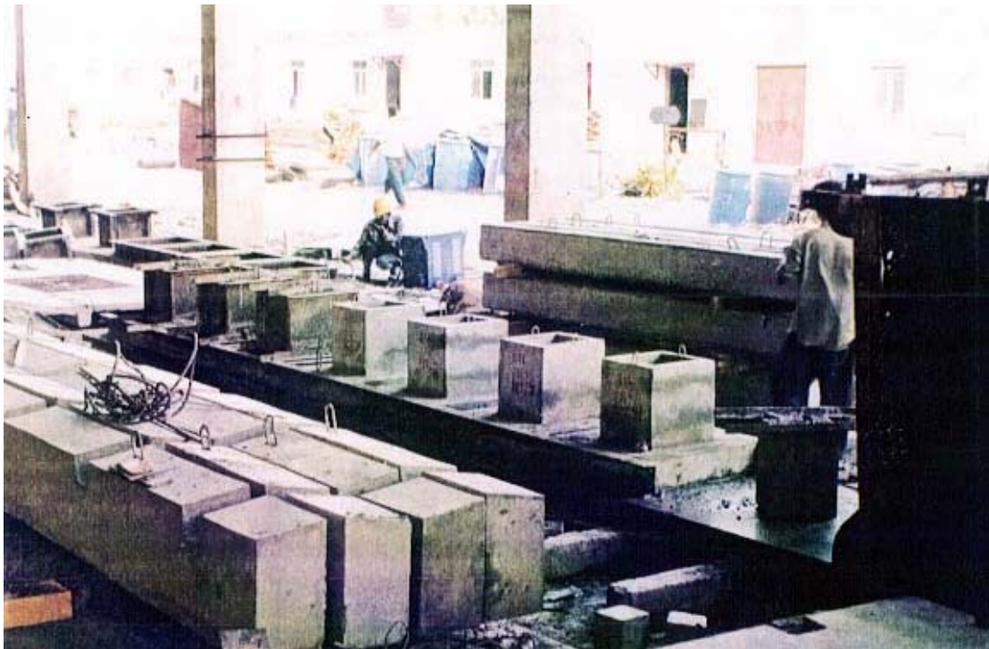
Finished Products: Beam, Footing & columns as on 30/12/01
