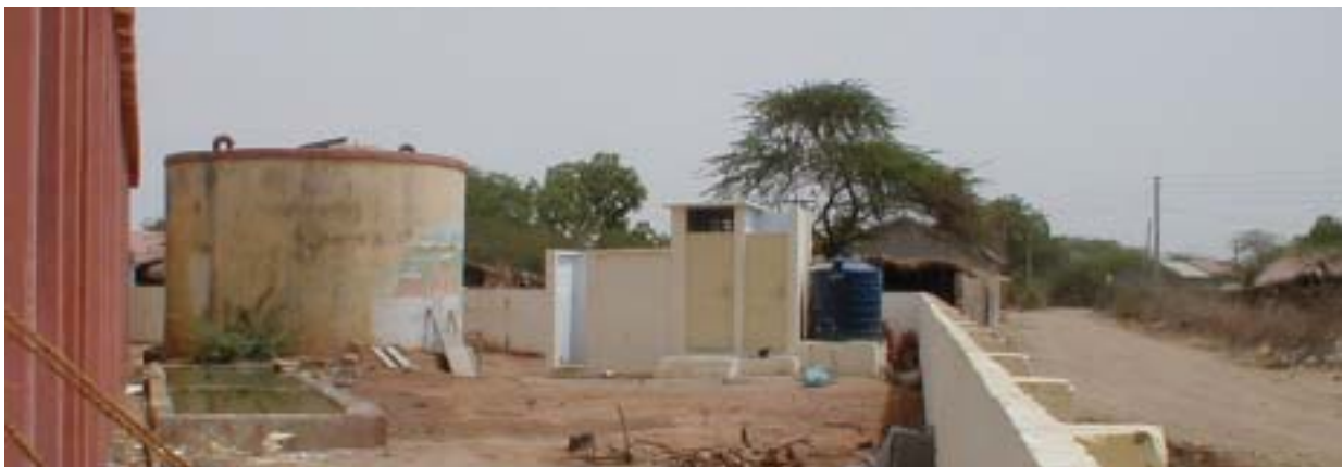
Sumarasar Sheikh Primary School Backyard Boundary Wall and Toilet Block (17/05/2002)
