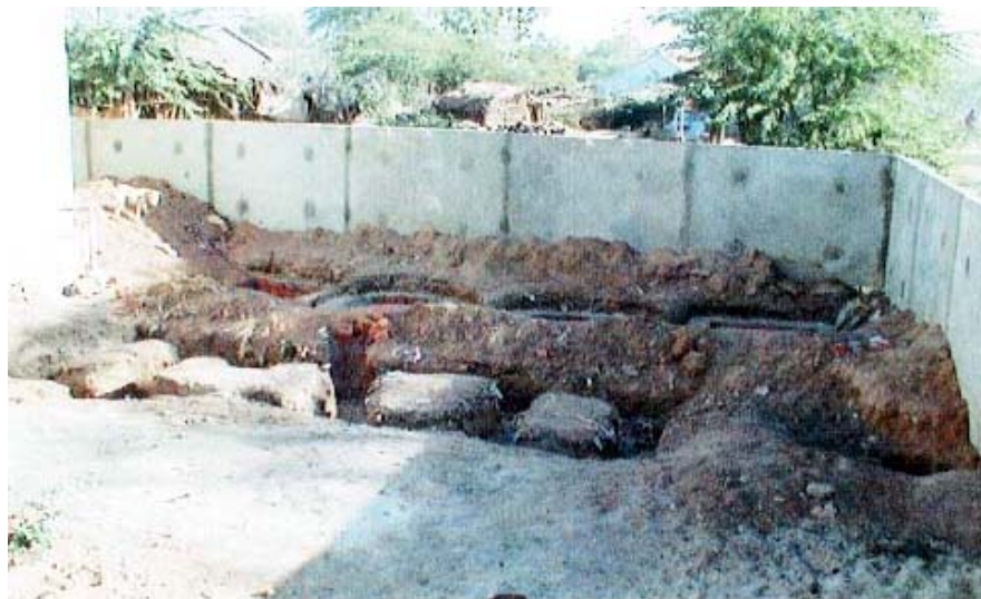
Sumarasar Sheikh Primary School Toilet Block (28/03/02)
