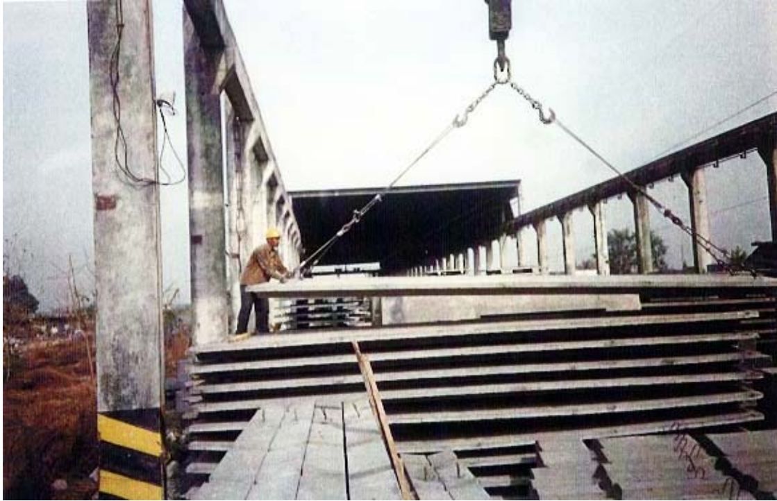
Stacking of Wall Panels 23/01/02
