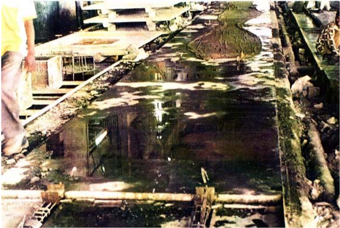
Curing In Progress Of Wall Panels as on 18/12/01
