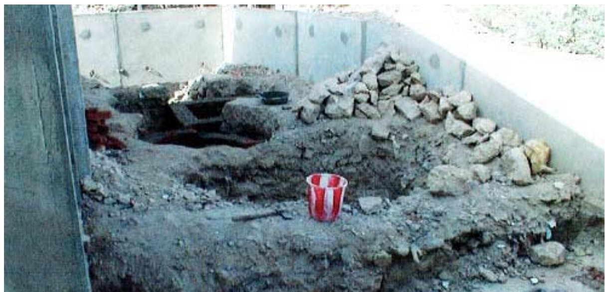
Mathak Primary School Toilet Block (27/03/02)
