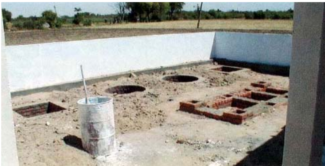
Dhamadka Primary School toilet Block (28/03/02)
