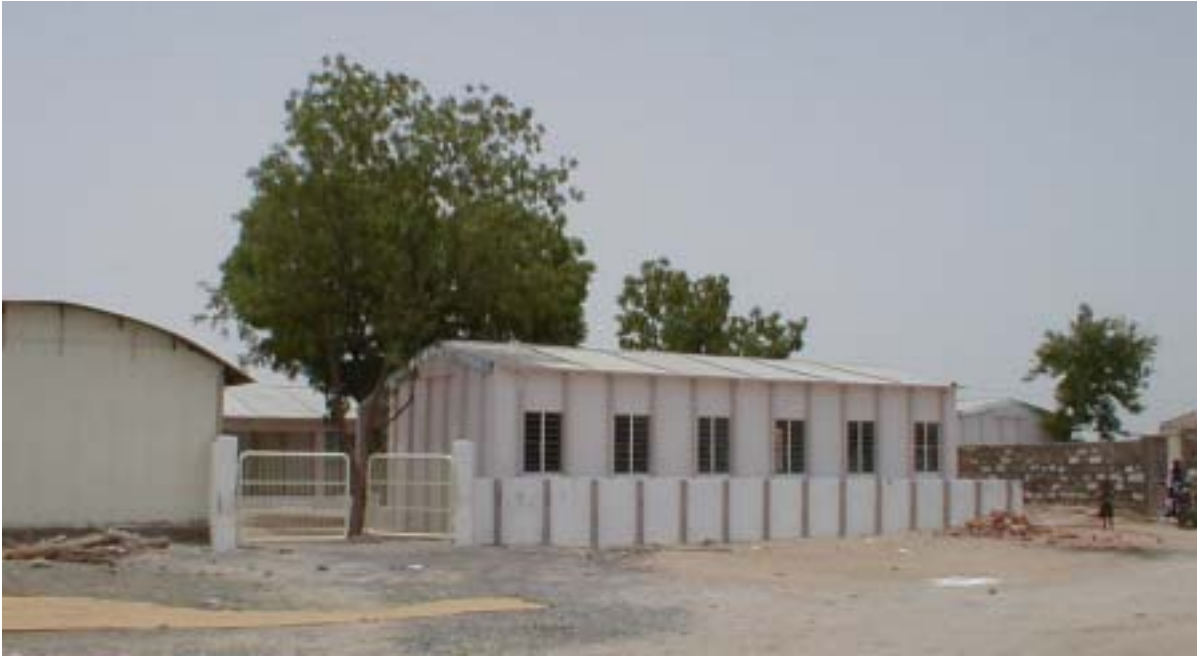
Dhamadka Primary School Front Side (17/05/2002)
