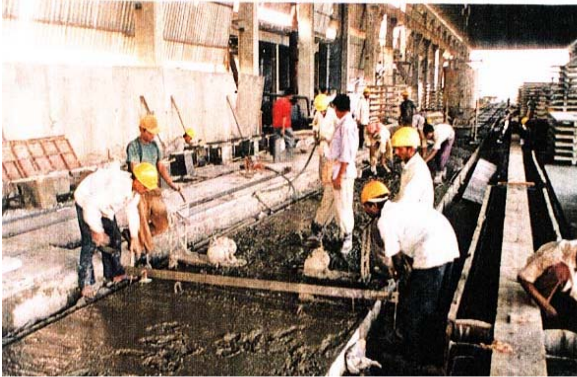
Vibrating In Progress Of Wall Panels as on 17/12/01
