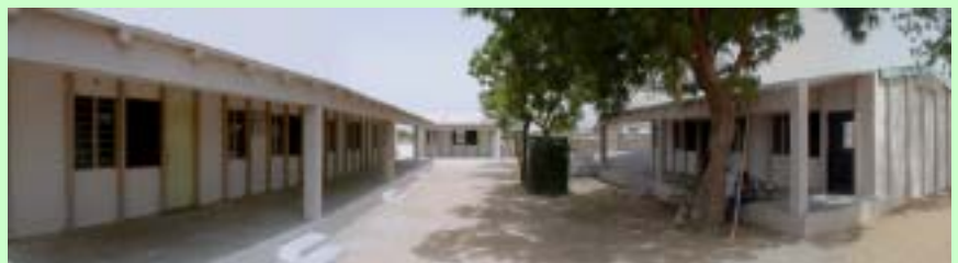
DHAMADKA PRIMARY SCHOOL
