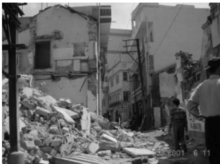
Fig.-1-1 Urban Area in Bhuj (June 11, 2001)
