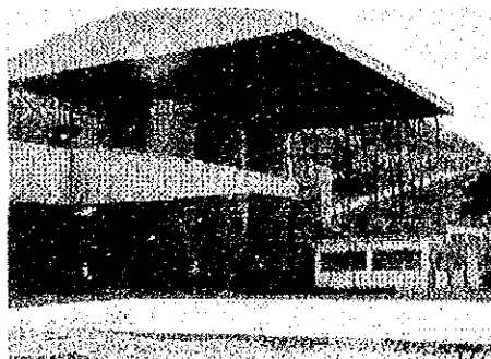
Waste Blending Facility
