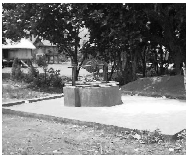
Photo 3 Dug well. Well constructed with apron and raised sides. This type could be improved with a handpump or small electric pump (Option 3)
