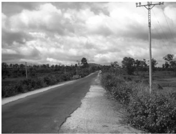
Photo 2 Thinly populated area (G4). Long pipelines increase cost and risk of leakage (Option 2)
