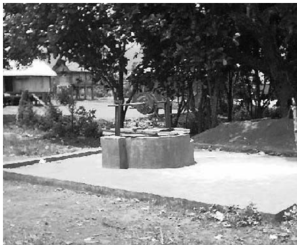
Photo 3 Dug well. Well constructed with apron and raised sides. This type could be improved with a handpump or small electric pump (Option 3)
