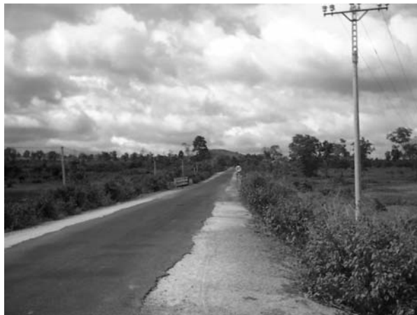
Photo 2 Thinly populated area (G4). Long pipelines increase cost and risk of leakage (Option 2)
