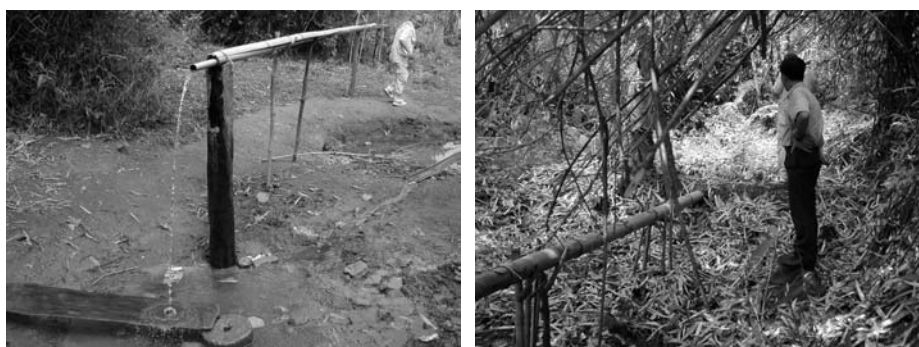
Left: Public piped water supply system is made of bamboo and woods at Dac Ui commune in Kon Tum province. A board and a stone are used for washing cloths. PVC pipe is recently used for reinforcement. Right: Water intake at spring
