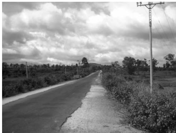
Photo 2 Thinly populated area (G4). Long pipelines increase cost and risk of leakage (Option 2)
