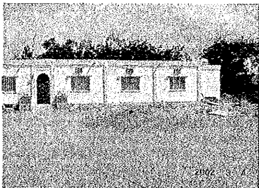
↑ (Photo-107) Existing facility within the proposed construction site
