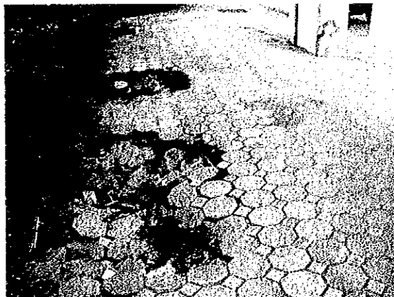
Figure 6-8 Collapsed Block Pavement dues to Poor Sand Compaction
