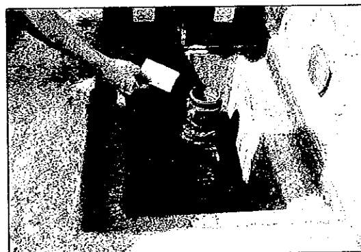
Figure 6.4.2 Underground Type Hydrant
