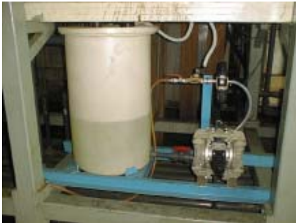
Diaphragm Pump for Rinsing Water Reuse
