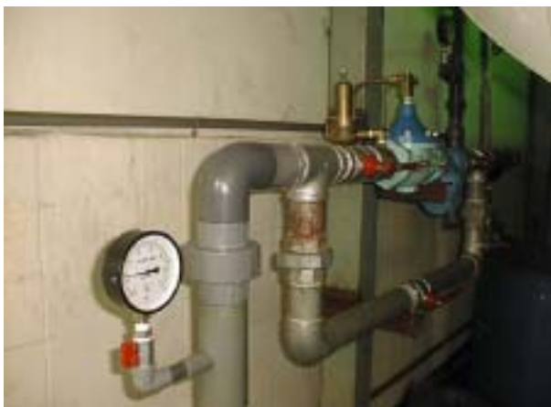
Pressure Control Valve to Control City Water Inlet Pressure
