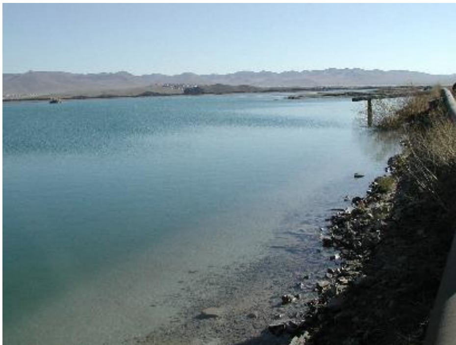
Nearby West Side Embankment
