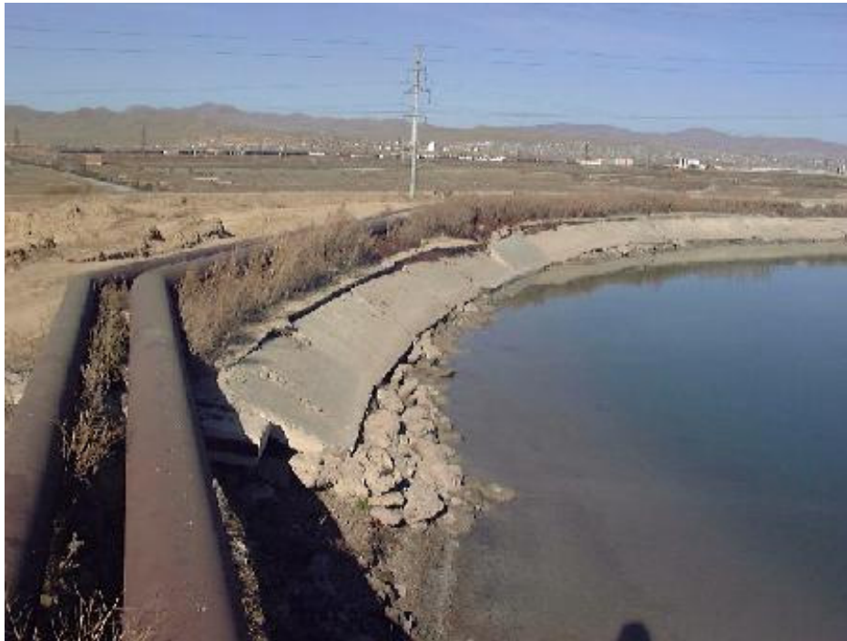
West Corner of the North Side Embankment
