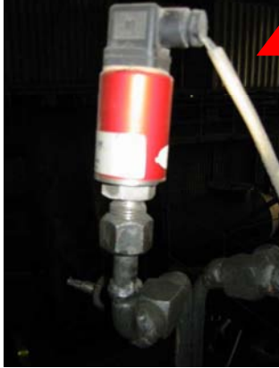
The pressure transmitter for turbine bearing
