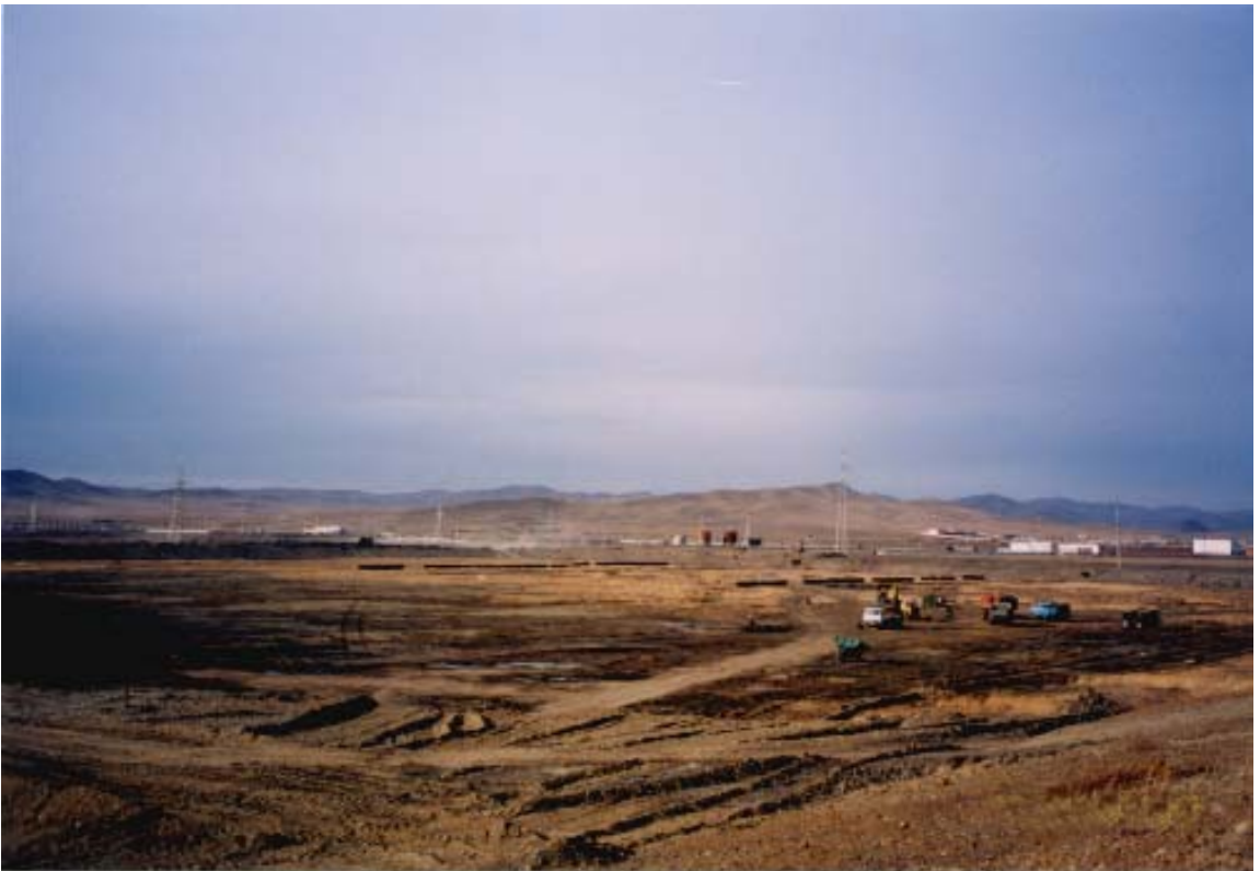
No.4 Ash Pond (Under Construction)
