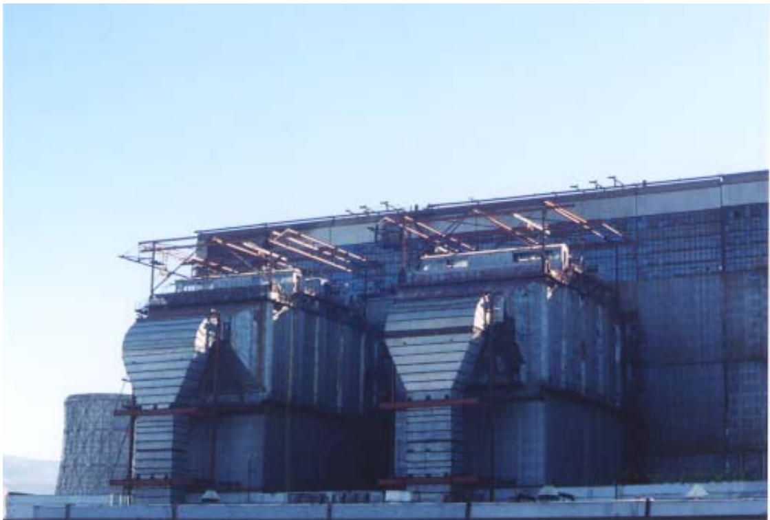
Electro Static Precipitator (ESP)
