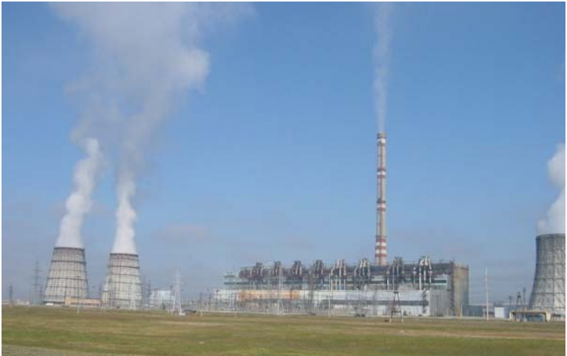
Power Plant General View
