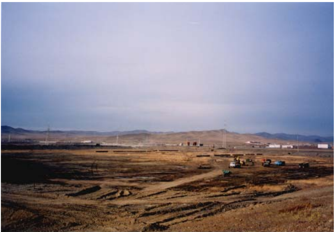
No.4 Ash Pond (Under Construction)
