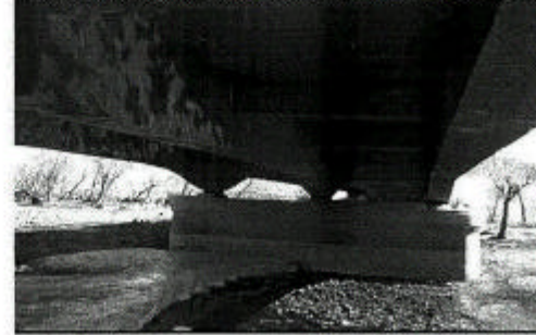
UB-Darhan 155.7km Girder width 50cm Constructed year 1950s, by Russian
