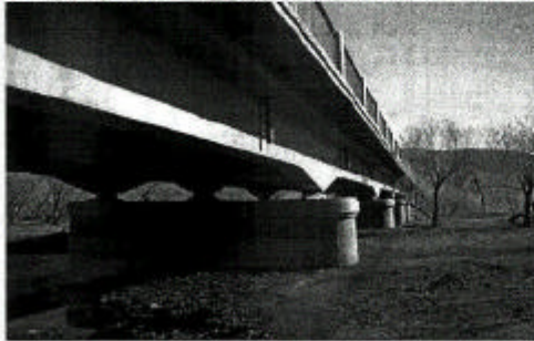
UB-Darhan 155.7km Continuous RC T Girder with Cross Beam
