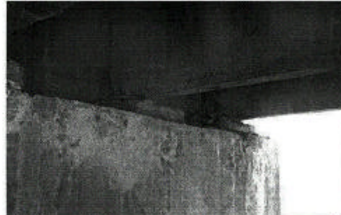
Ikh Tenger Bridge in UB, Girder end broken, crack re-bars exposed Constructed 1994
