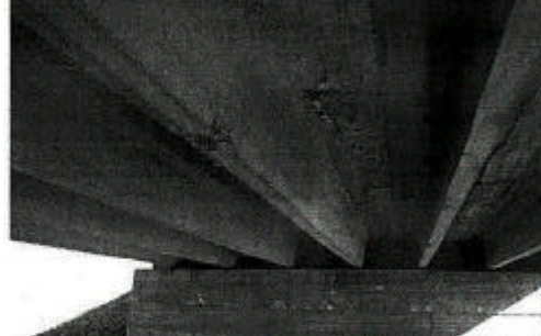
UB-Darhan 91.0km Exposed re-bars, slab defects Insufficient slab. Constructed by Gan guur cont.1999
