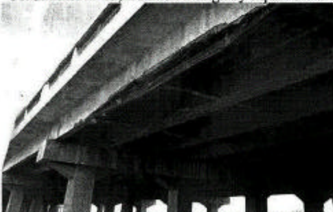
Enkhtaaivan Railway FO in UB, with cross beam Completely exposed re-bars, Constructed 1961
