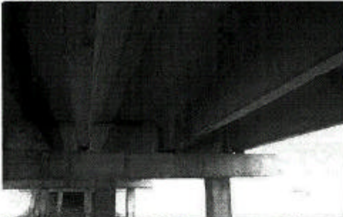
Nalaikh-Erdene RC T Girder without cross beam Repaired defects part by mortar
