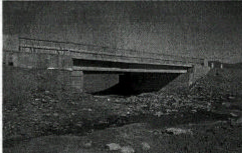
UB-Darhan 91.0km RC T Girder without Cross Beam Length 18m, Carriageway width 9.5m(Bor nuur river)
