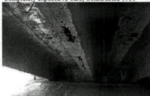
Dambadarjaa Bridge in UB, Exposed re-bars, slab lime leaking, Constructed 1995 (Selbe river)
