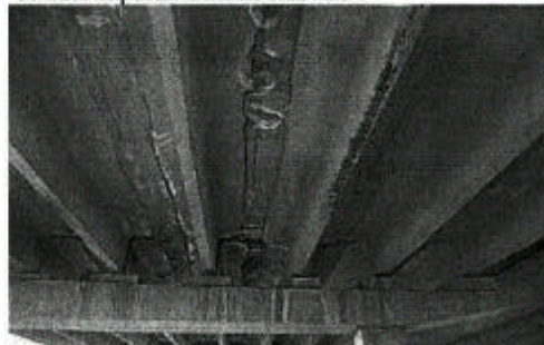
Gurvaljin Railway FO in UB, without cross beam Girder re-bars exposed, constructed 1989
