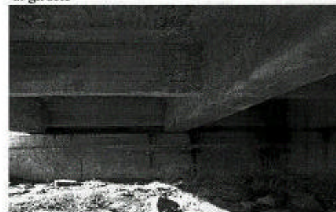
UB-Darhan 38.7km RC T Girder, L=8.7m, Carriage width 8.8m Constructed year 1950s by Russian Width of girder: 40cm
