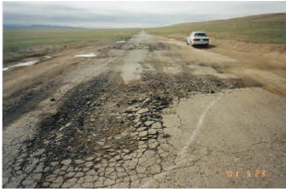
Photograph 8-3-1 Alligator Cracks
